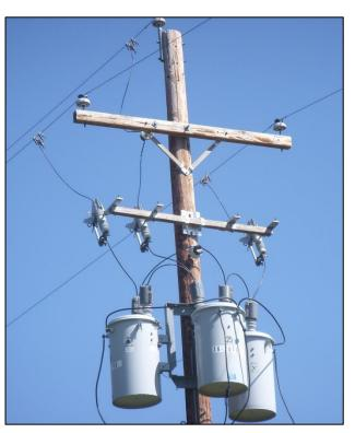
Retrofitted pole with equipment (transformers, cutouts, arresters) and avian-framed crossarm
