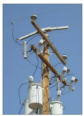
Retrofitted pole with equipment (transformers, cutouts, arresters) and insulator cover
