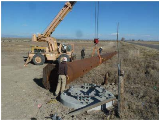
Setting structure on foundation
