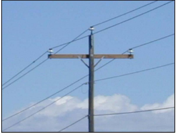
Three phase tangent, 10-foot arm ( Avian-safe construction )
