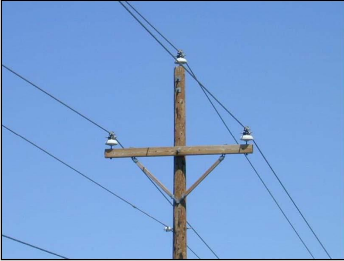
Three phase tangent, 8-foot arm ( Avian-safe construction )
