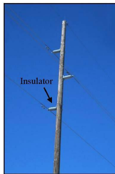
Post-mounted insulators
