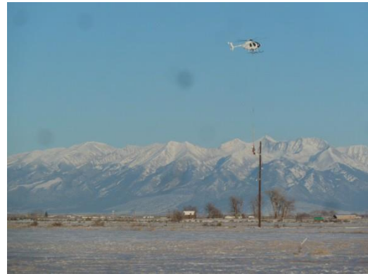
Conductor stringing with helicopter
