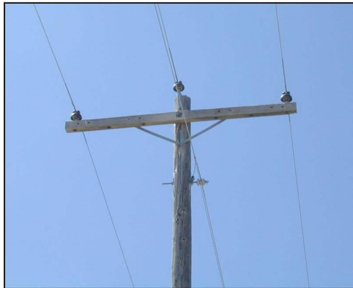
Three phase tangent, 8-foot arm ( Avian-safe construction )
