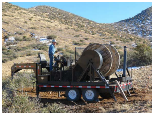
Cable reel/pulling location: 8 – 10 feet wide, 25 – 40 feet length, and weight 10 – 20 tons.
